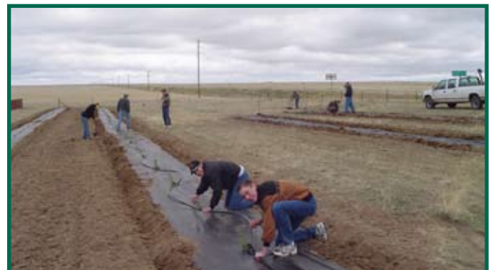
Drip irrigation installation for newly planted trees.
